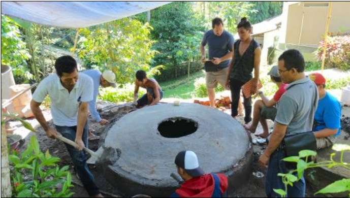
Indonesian farmers build a cistern at the Bali Appropriate Technology Institute (BATI)
